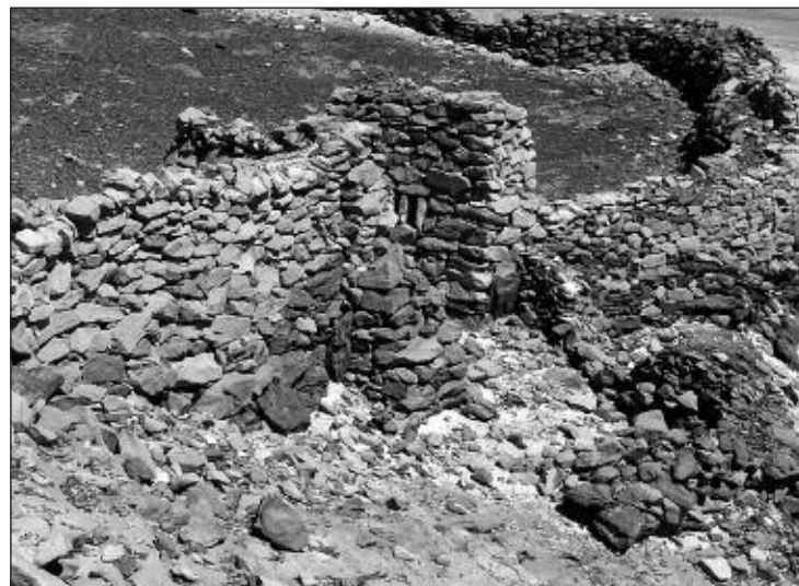
Fig. 5. Gate passage on the east side of main fort with partly collapsed structure at entrance and possible bolt hole. Height 2.8 m, width c. 2.0 m.
