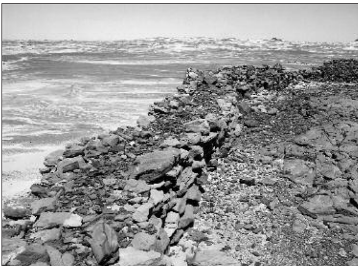
Fig. 4. Close-up of wall showing sandstone masonry and rubble-filled core. Width c. 1 m.
